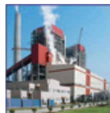
7 - LONG AN POWER PLANT (1200MW)
