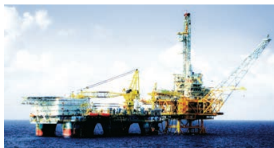
PV DRILLING V
