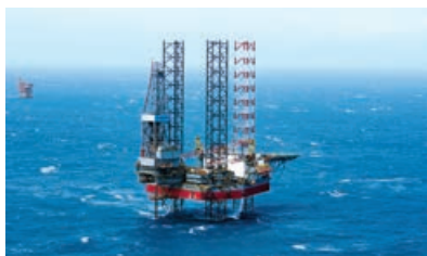
PV DRILLING I
