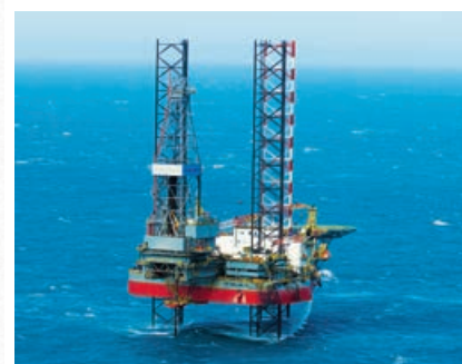
PV DRILLING II
