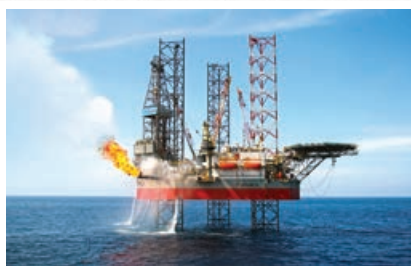
PV DRILLING III
