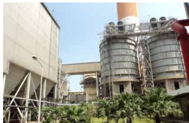
Pha Lai Thermal Power Plant
