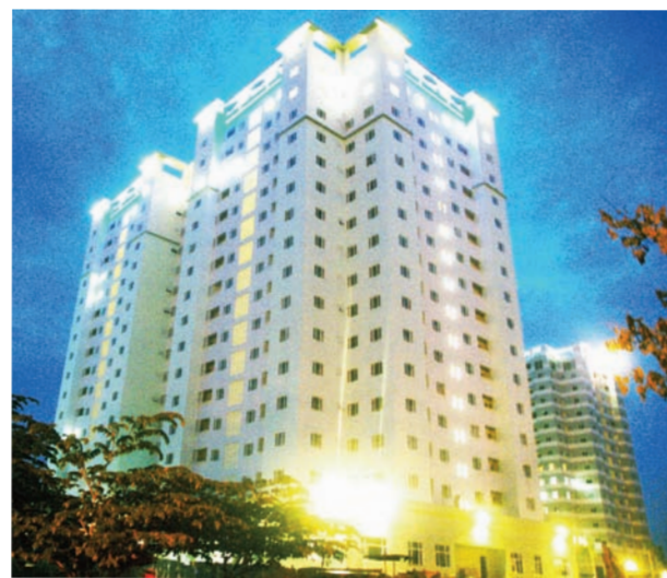
Nhat Lan 3 Apartment Building
