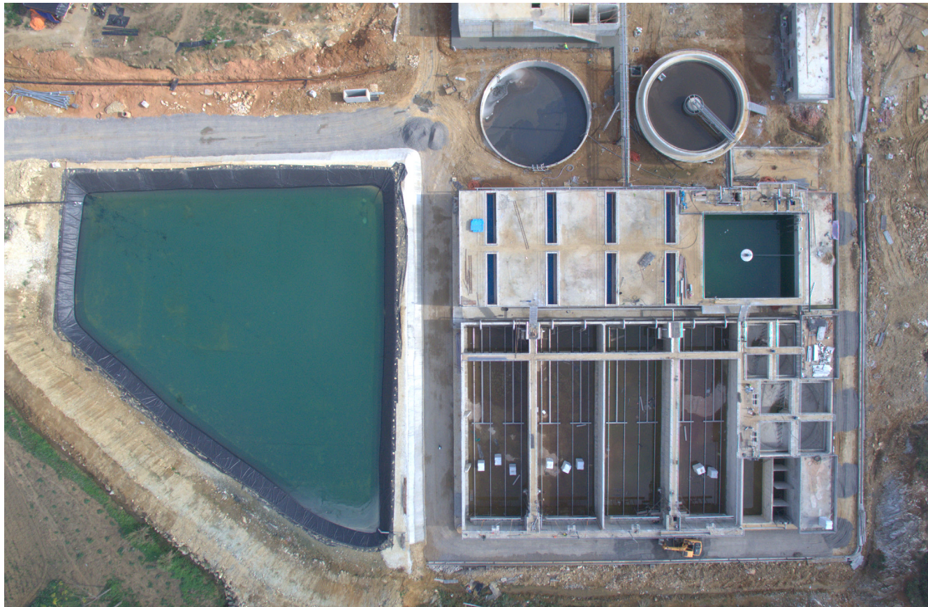
Masan Nutri-Farm's waste treatment plant in final stage of construction
