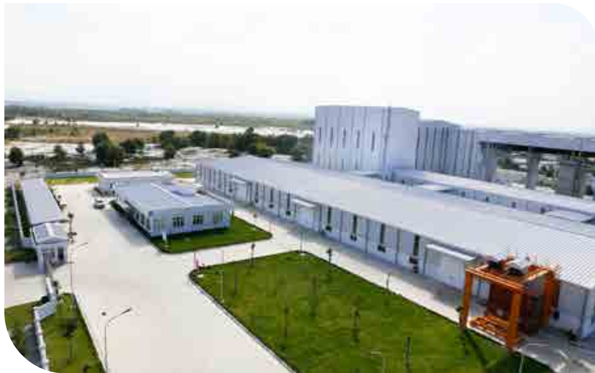
Overview of the Phenikaa Hue plant
