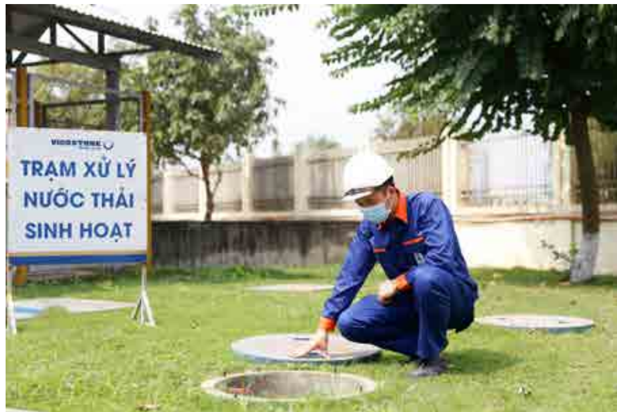
Wastewater treatment station
