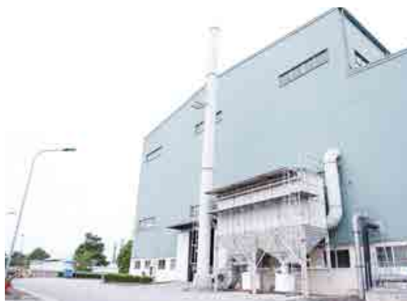
Dust treatment system in Vicostone's Plant
