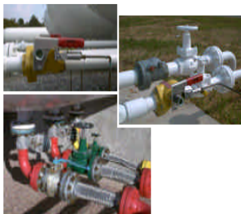
Misc. components of typical tank trim and ESVs
