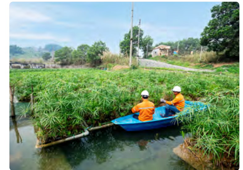
Hundreds of floating cyperus rafts (Thuy truc) at the biological filtration area near discharge point DP2
