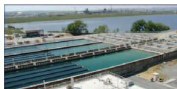
5 - KIEN LUONG WATER PLANT (200,000 m /day) 7 - LONG AN WATER PLANT (600,000 m /d ) 3 - HA NAM WATER PLANT (100,000 m /day)
