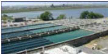
5 - KIEN LUONG WATER PLANT (200,000 m /day) 7 - LONG AN WATER PLANT (600,000 m /day)
