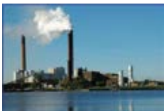
5 - KIEN LUONG POWER COMPLEX (4400/5200 MW)
