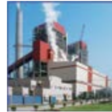
7 - LONG AN POWER PLANT (1200MW)
