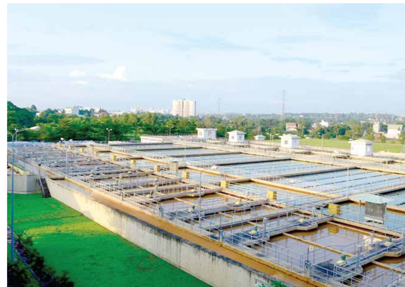
B.O.O Thu Duc Water Plant
