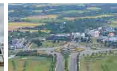
WATERPOINT COMMERCIAL 📍 Bến Lức, Long An
