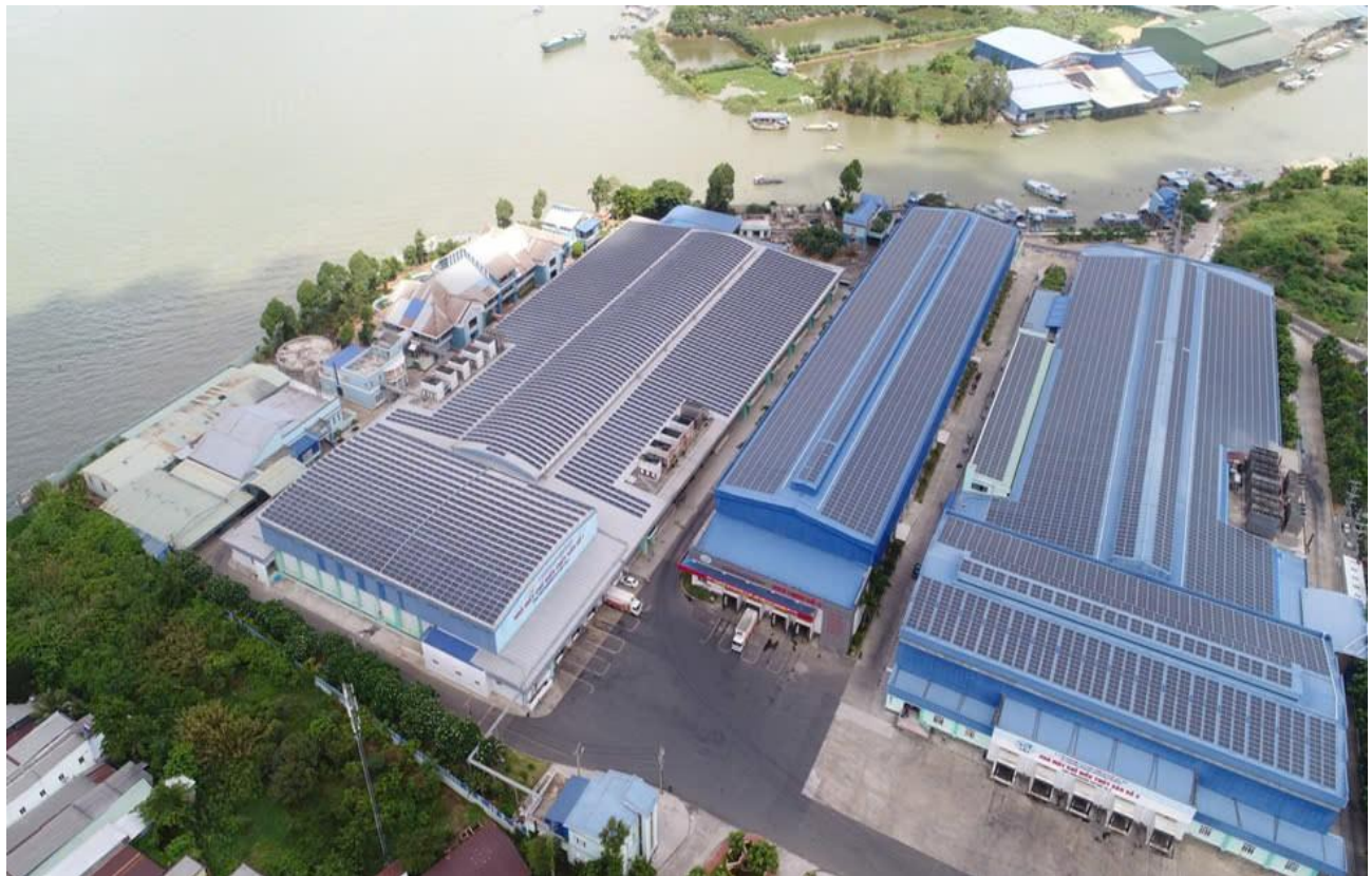
Solar power system on the roof of a seafood processing factory.
