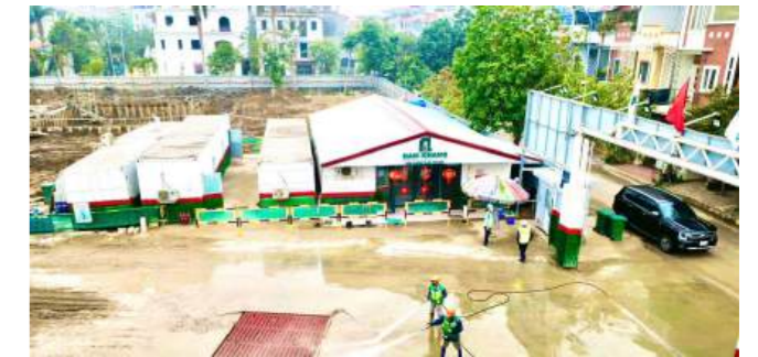
Construction site An Dong, Hai Phong
