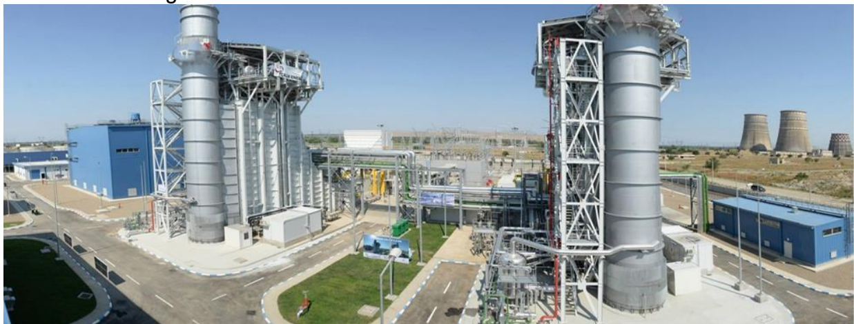
Project of upgrading capacity, performance for Phu My 1 TPP
