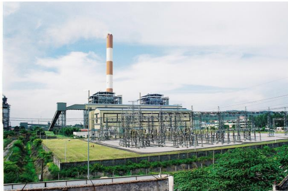
Retrofitting for equipment improvement Pha Lai TPP
