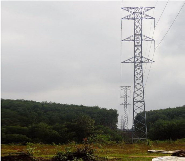
220kV An Khe - Quy Nhon T/L circuit 2, combined improving circuit 1
