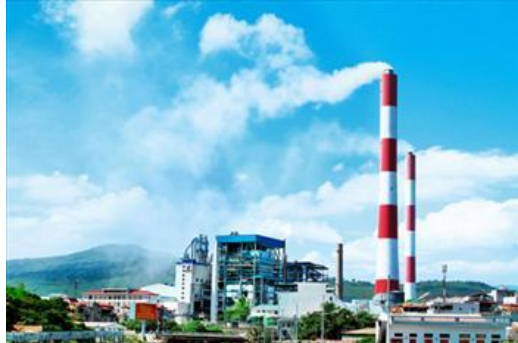
Transferring FO – DO system Uong Bi TPP
