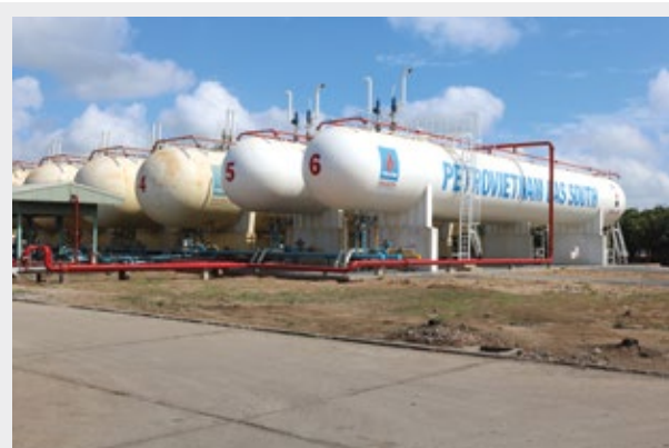
Can Tho LPG storage and extraction station (with the capacity of 1,600 MT) provides industrial LPG and residential LPG for South-western region.
