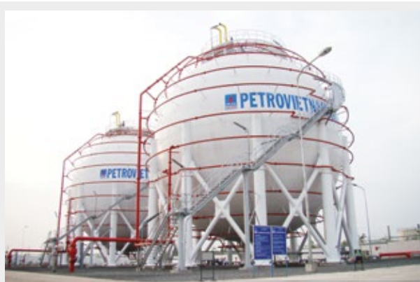
LPG Go Dau storage, Dong Nai Province (with the capacity of 4,000 MT) provides industrial LPG for South-eastern region.
