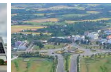
WATERPOINT COMMERCIAL 📍 Bến Lức, Long An
