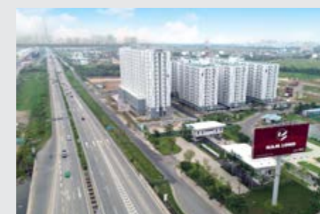
EHomeS - Phu Huu 📍 District 9, Thu Duc - 1,240 units
