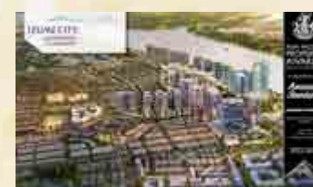
Mixed Use Development Vietnam for Izumi City (Bien Hoa City, Dongnai Province)
