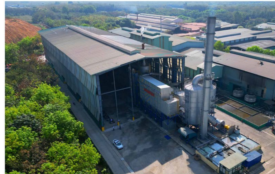
NAM BINH DUONG INTEGRATED SOLID WASTE TREATMENT COMPLEX
