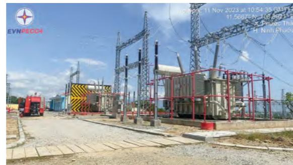
220kV Phuoc Thai Substation expansion
