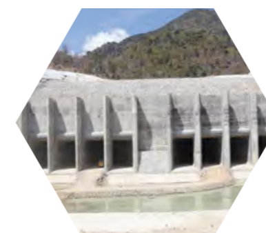
Bac Ai Pumped Storage Hydropower Plant
