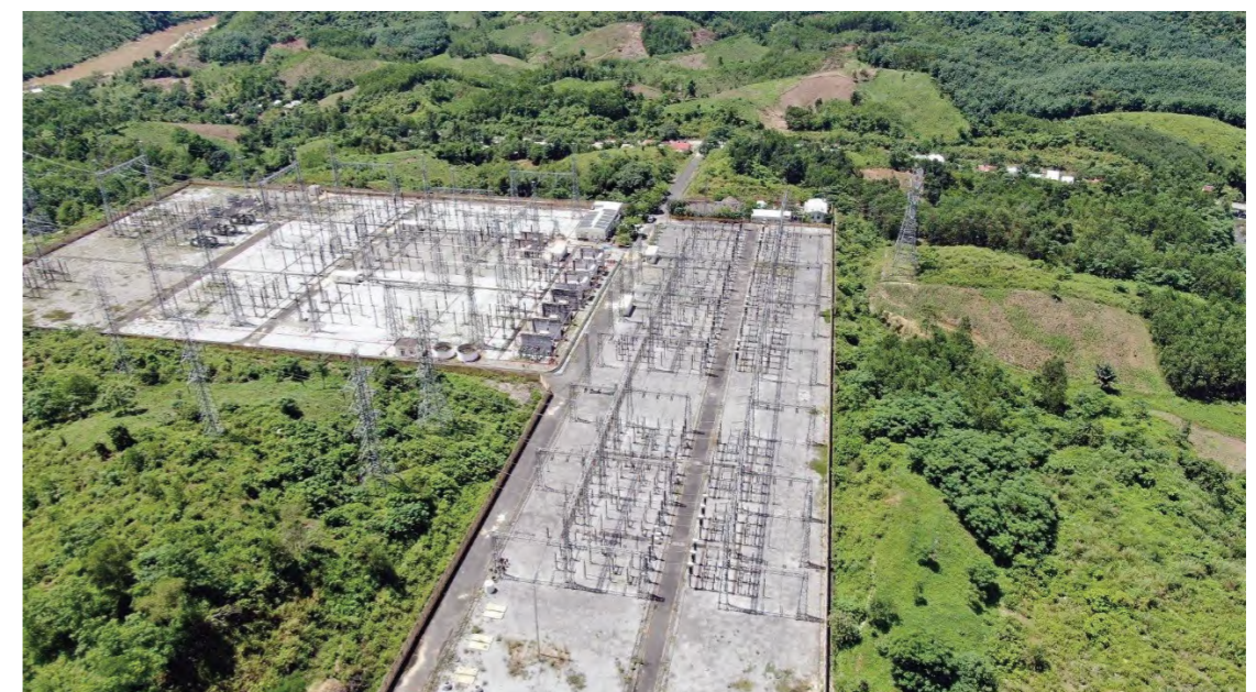
Supervision consulting for the 500kV Monsoon - Thanh My transmission line
