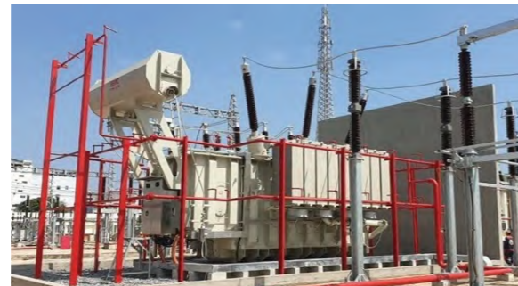
Increase the capacity of 500kV Quang Ninh Substation project
