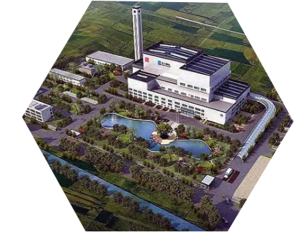
Bac Giang Waste Power Plant
