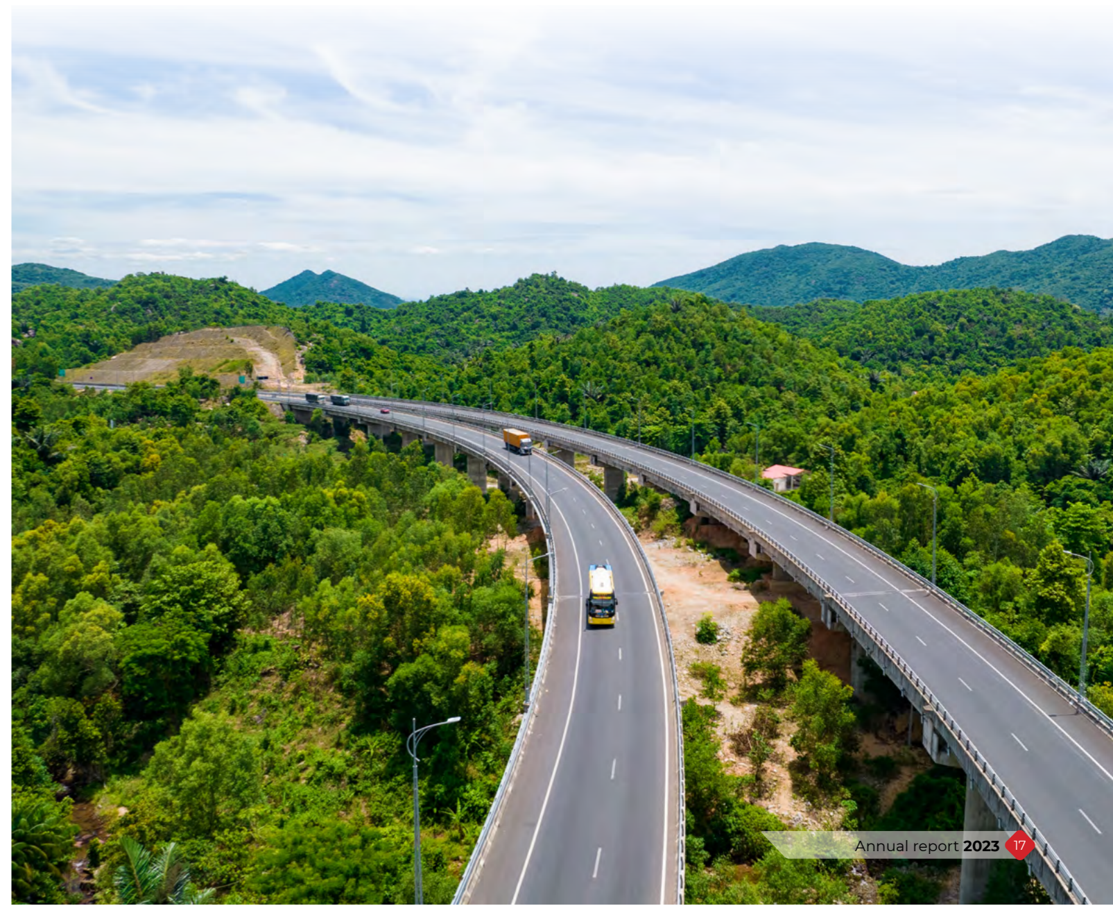
Deo Ca tunnel project
