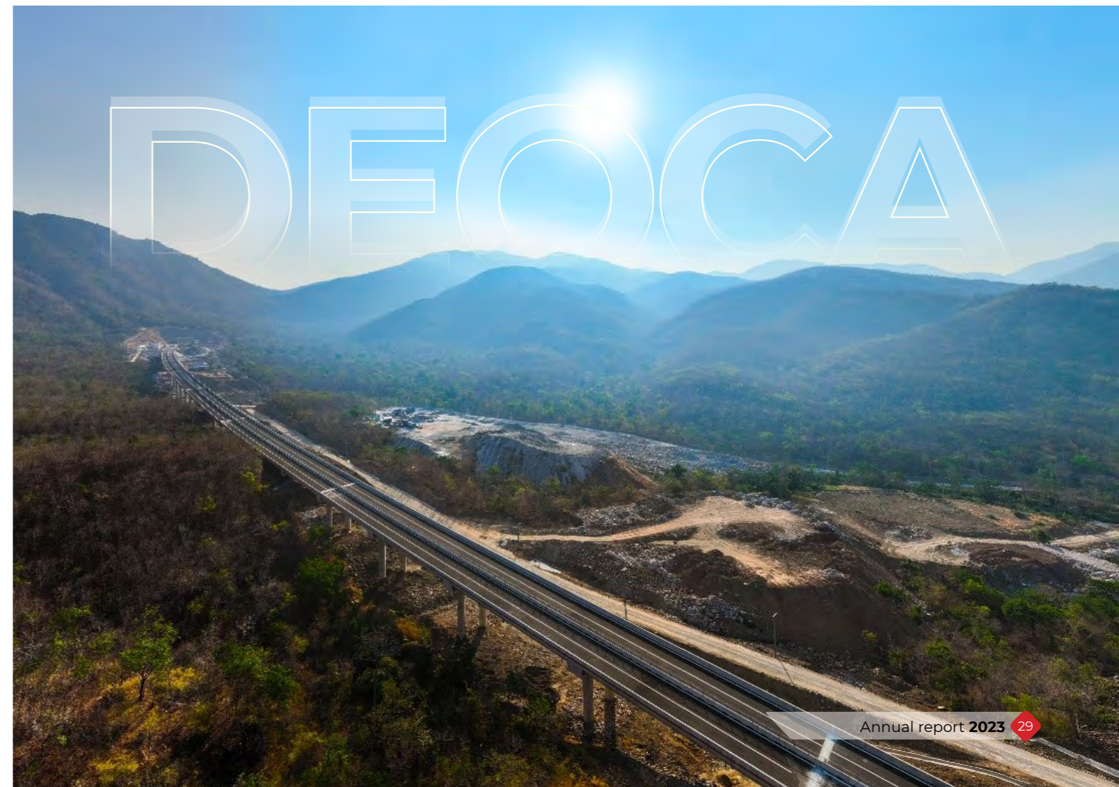
Cam Lam – Vinh Hao Expressway Project
