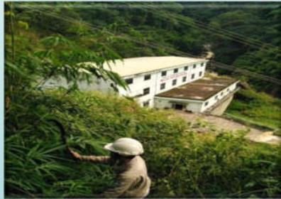
Clean-up and Landscape Maintenance at Dak Pone Hydropower Plant.
