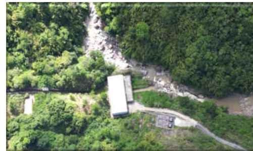
The landscape of Đăk Pône Hydropower Plant.
