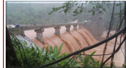
The floodwater on the Đakrông River rose above the free overflow
