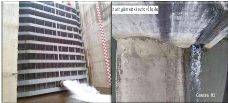
Ensuring environmental flow for the downstream area of Đa Krông 1 Hydropower Plant Dam
