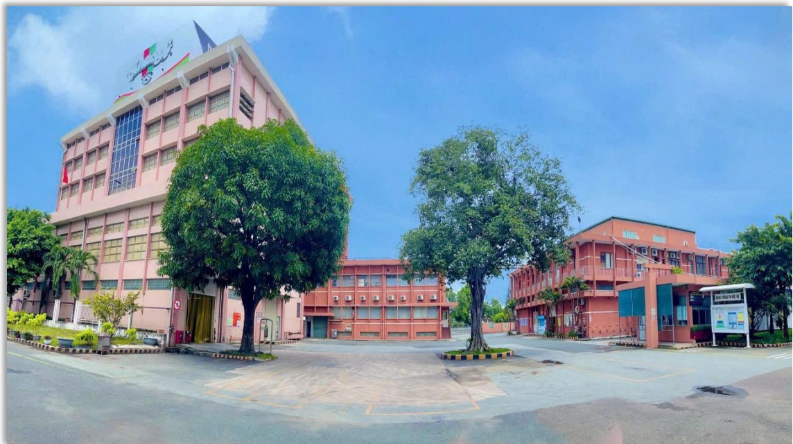
Factory premises at Bien Hoa 1 Industrial Park, An Binh Ward, Bien Hoa City, Dong Nai Province
