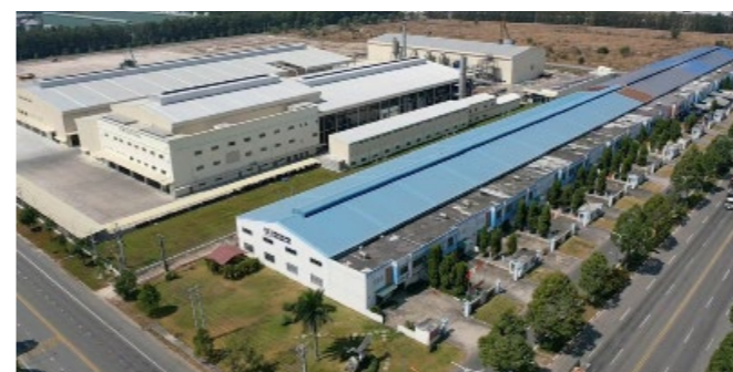
Bau Bang Industrial Park Expansion Project
