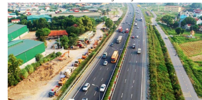
Ho Chi Minh City - Thu Dau Mot - Chon Thanh Expressway Project
