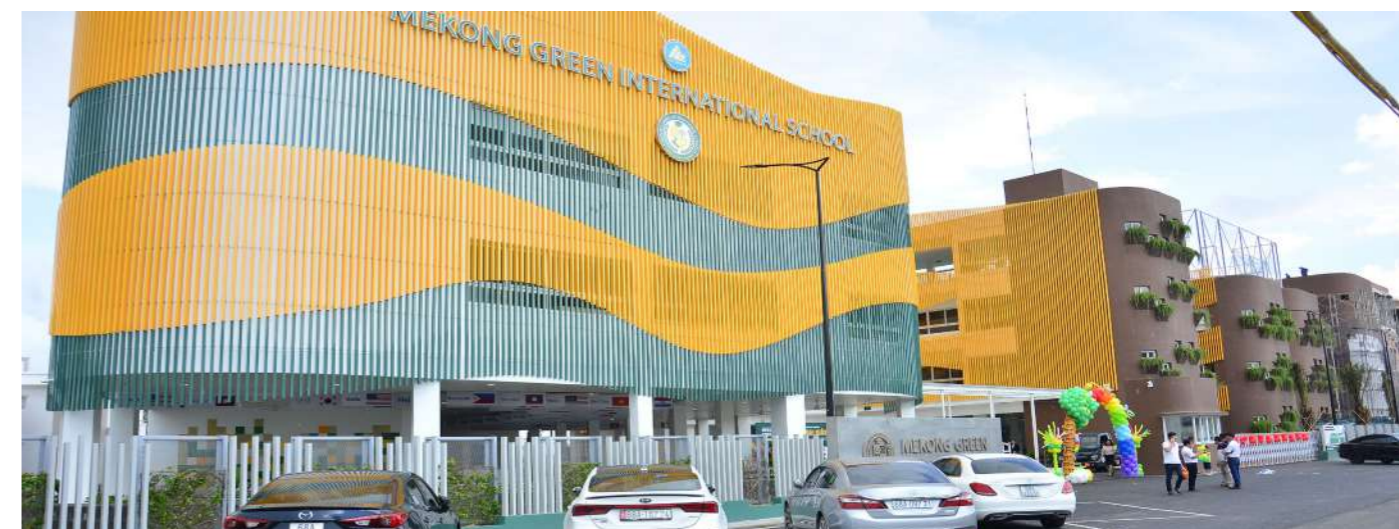
A corner of the investment project to build the Mekong Green International Kindergarten and Primary School
