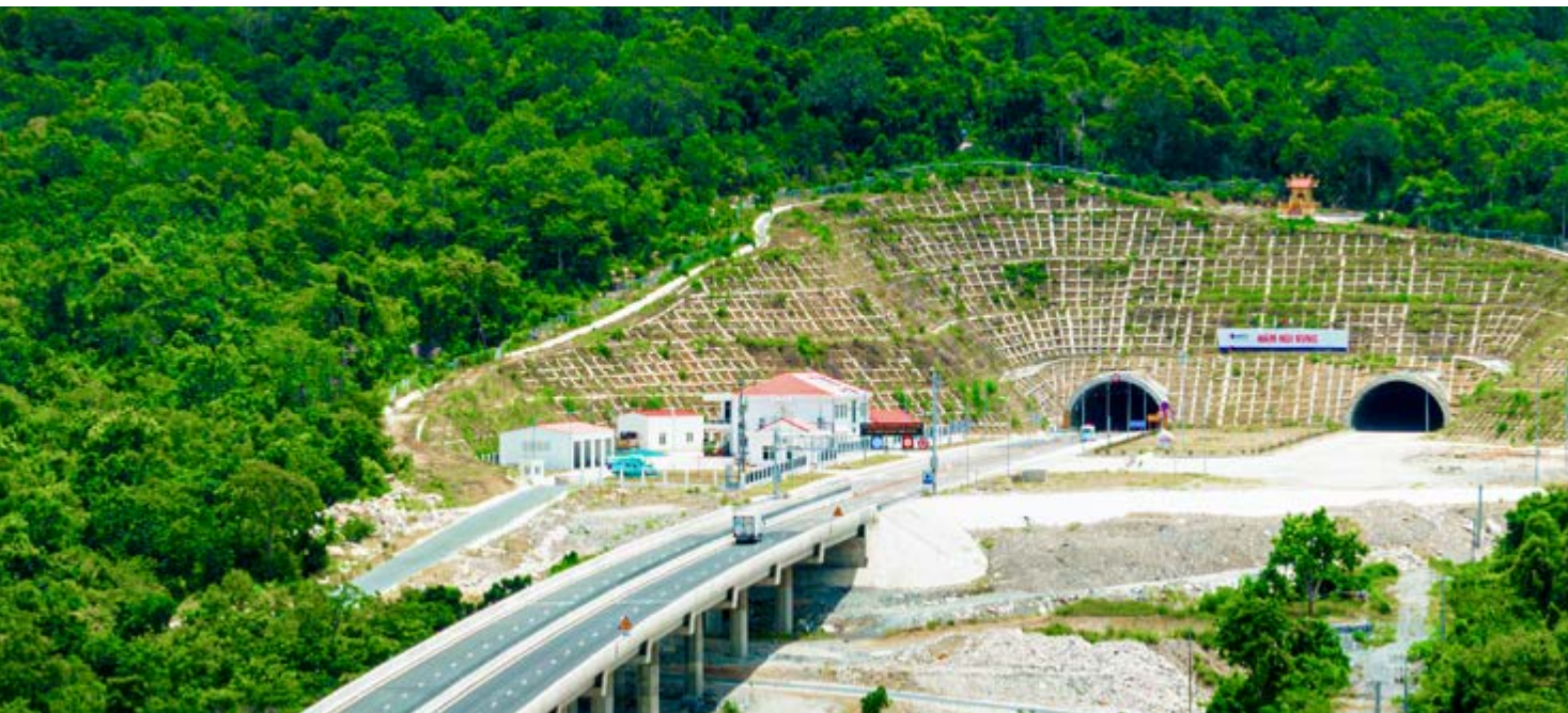
Mountain tunnel on expressway project Cam Lam - Vinh Hao
