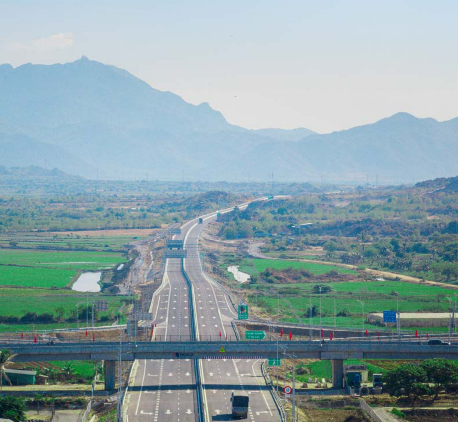
Cam Lam - Vinh Hao Expressway Project
