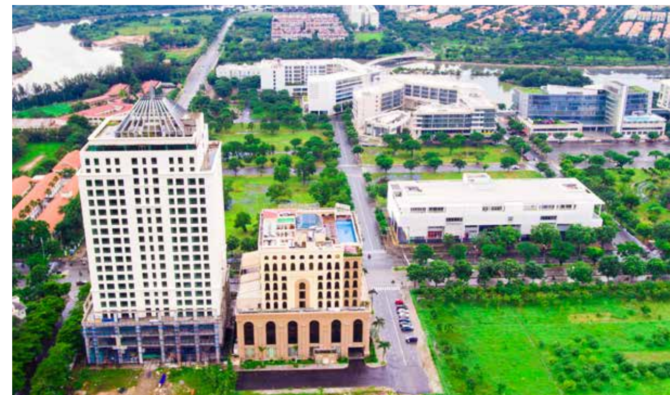
COMMERCIAL BUILDING GOLDEN KING
