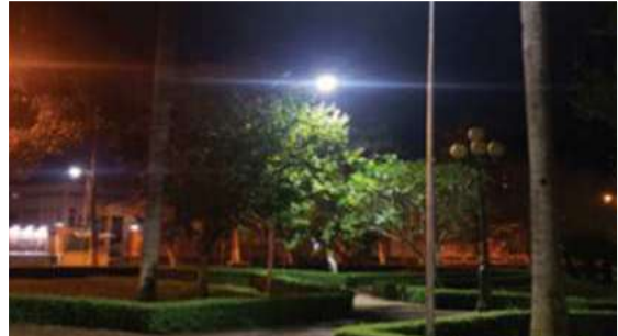
Solar Lighting at Dong Nai Military Command
