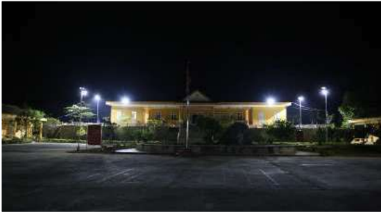
Solar Lighting at Chieng Tuong Border Guard Station - Yen Chau - Son La
